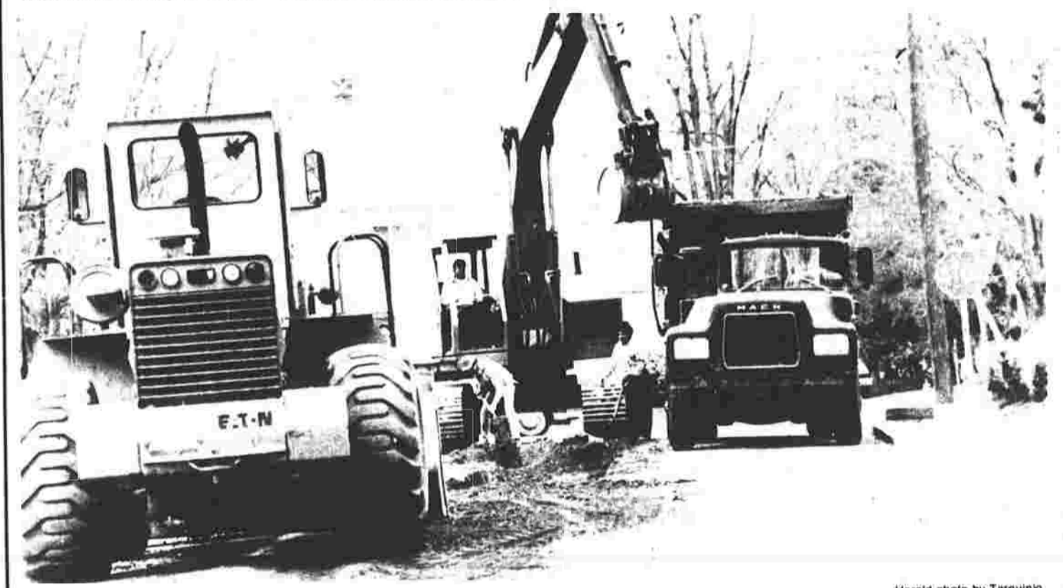
Porter project under way
